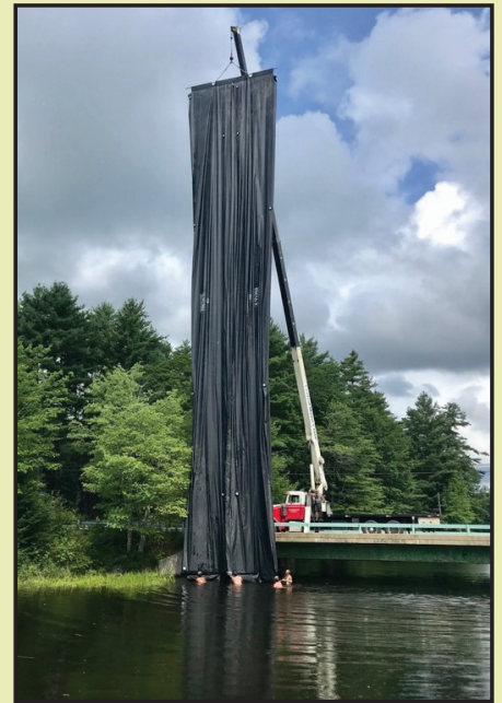
Coffer dam being positioned
